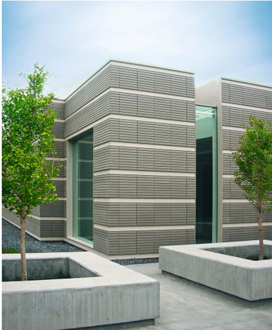
Terra-cotta panel façade, GoettschPartners ,
