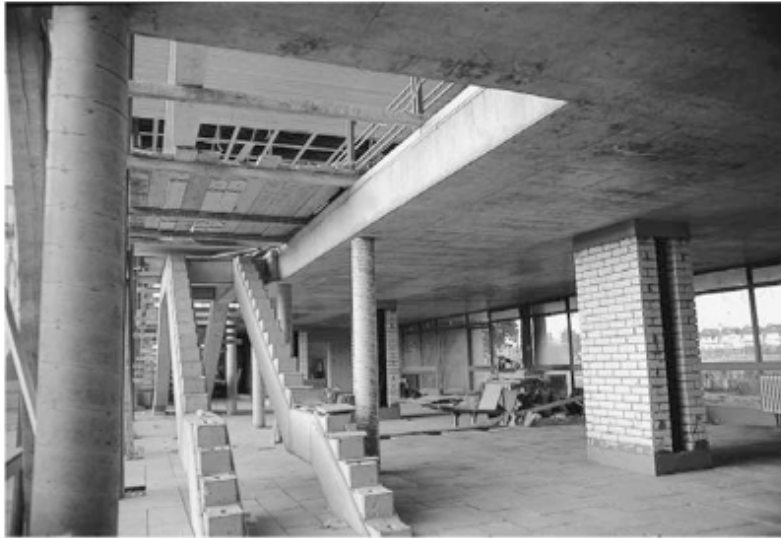
Figure 8.3b Pre-cast beam stair prepared for tread fixing
