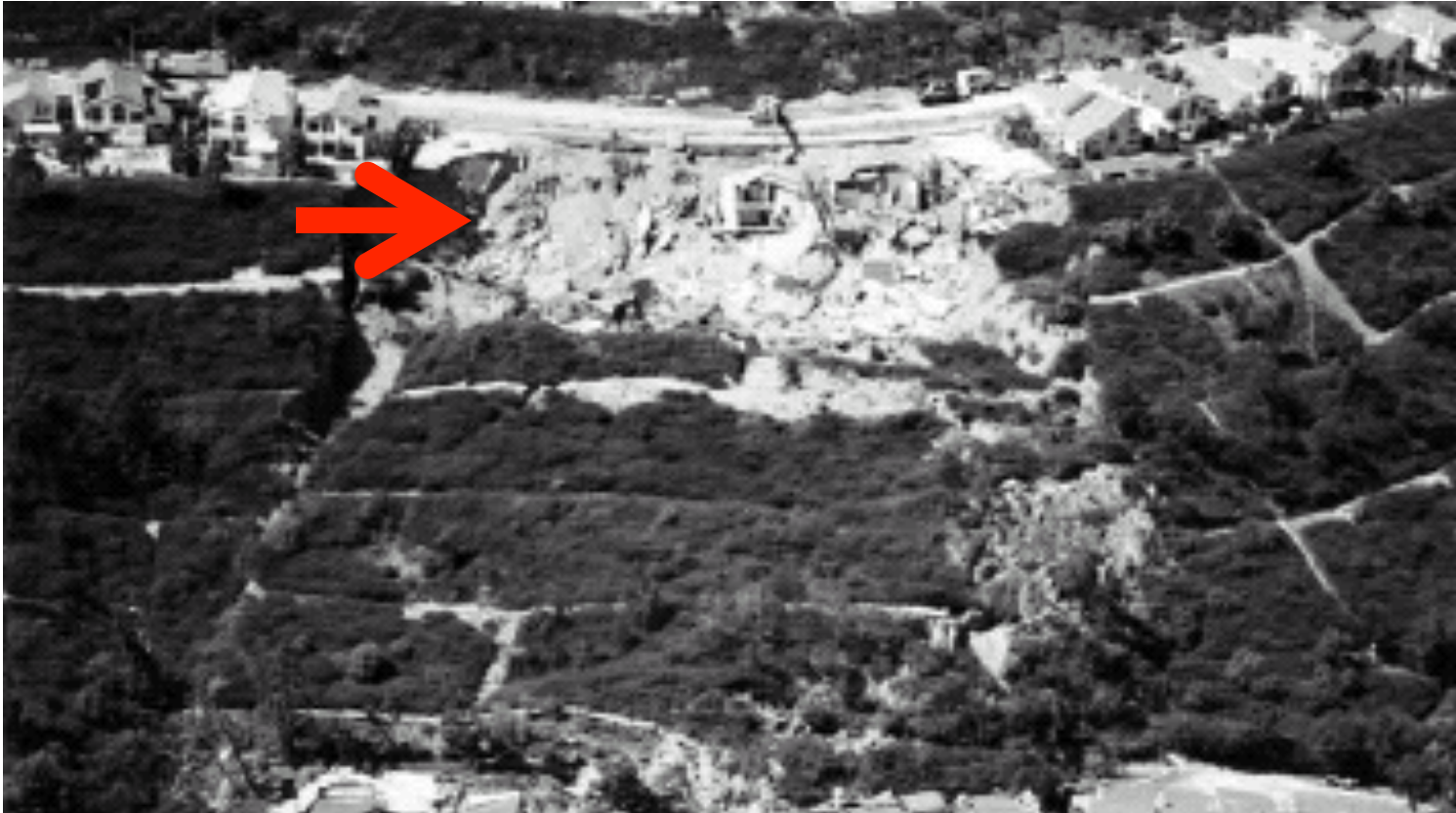
The Laguna Niguel landslide March 19, 1998
