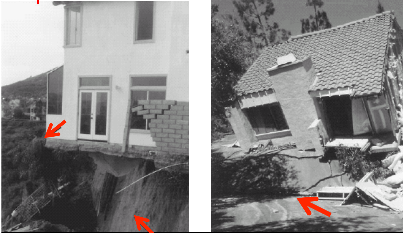
The Laguna Niguel landslide March 19, 1998
