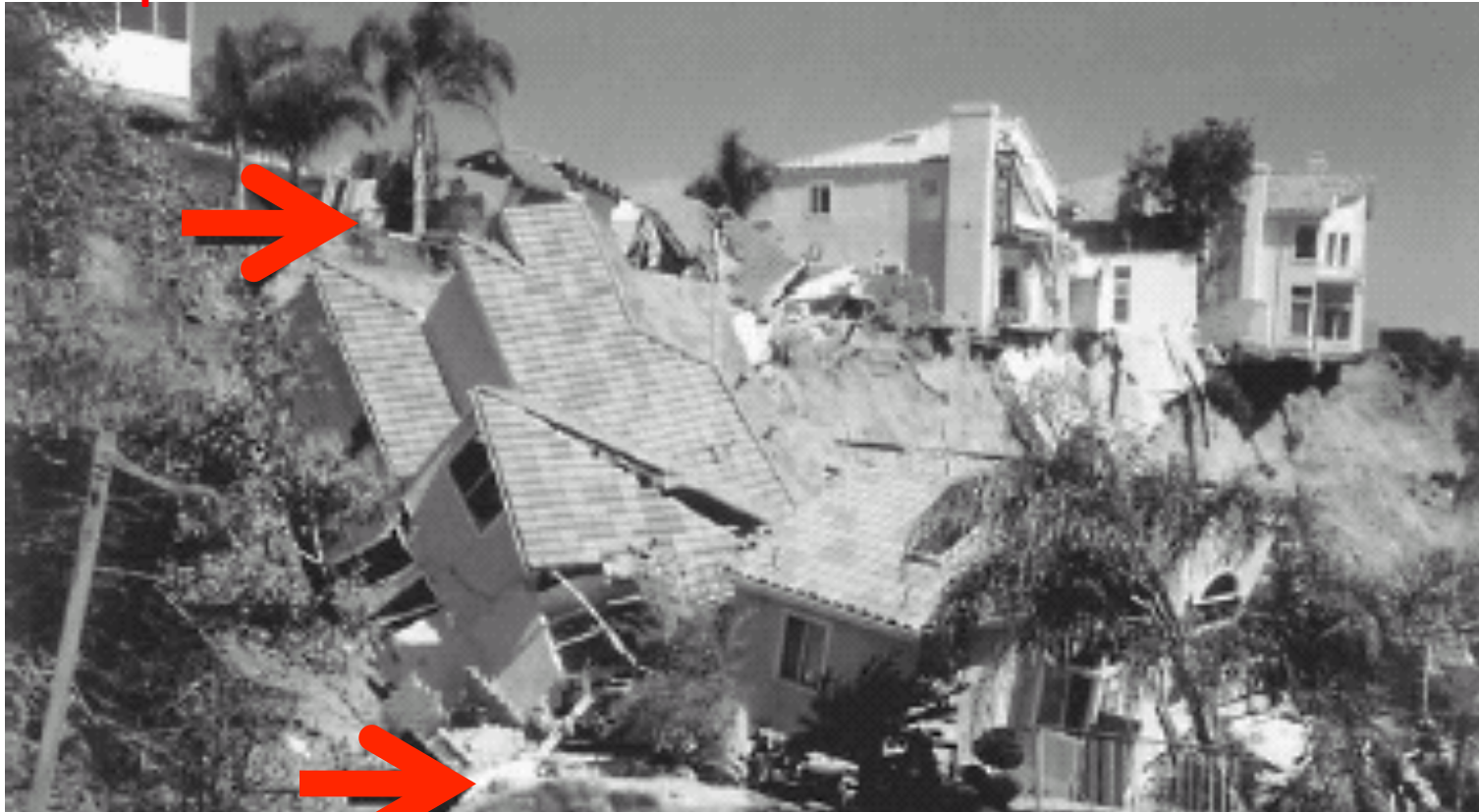
The Laguna Niguel landslide March 19, 1998
